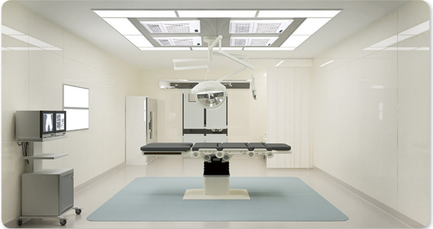
4 laminar flow air purifiers in operating room
